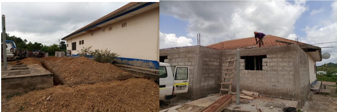
11. Completion of the Phase II of the Paving of the Floor of the Bogoso Market
